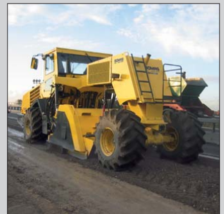
Recycling applications, with optional injection of bitumen emulsion or foam bitumen.
