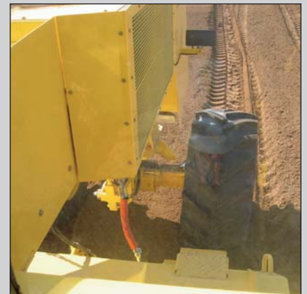
Excellent view over the entire working area and treated material.
